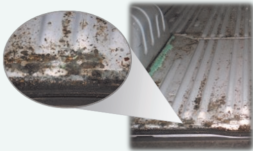
Formation of mould under standard wooden floors.
